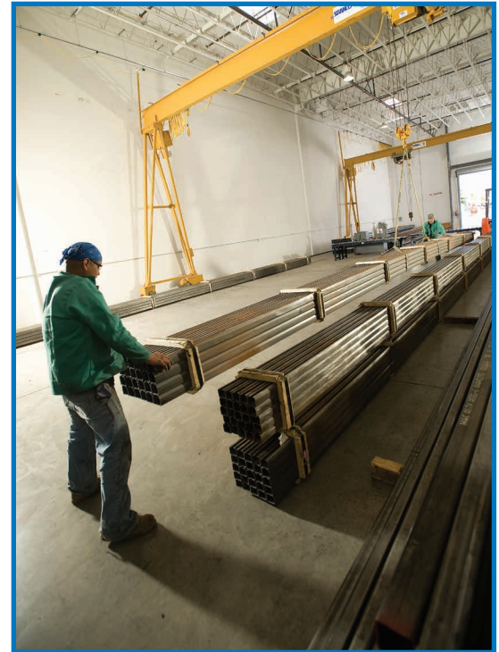
Workers using two Motorized Spanco PF Gantry Cranes to load and transfer steel bundles.
